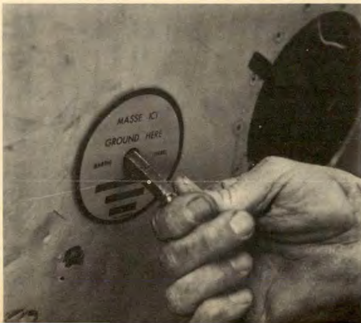
Standard grounding system, plug and receptacle such as shown here in photo of C-141. Program seeks to standardize grounding among military services, civilian agencies, foreign nations.
